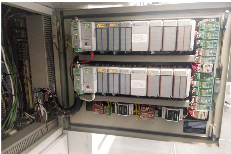
The Finished Installation
